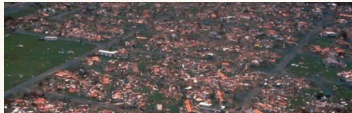
The devastation left behind by Hurricane Andrew
