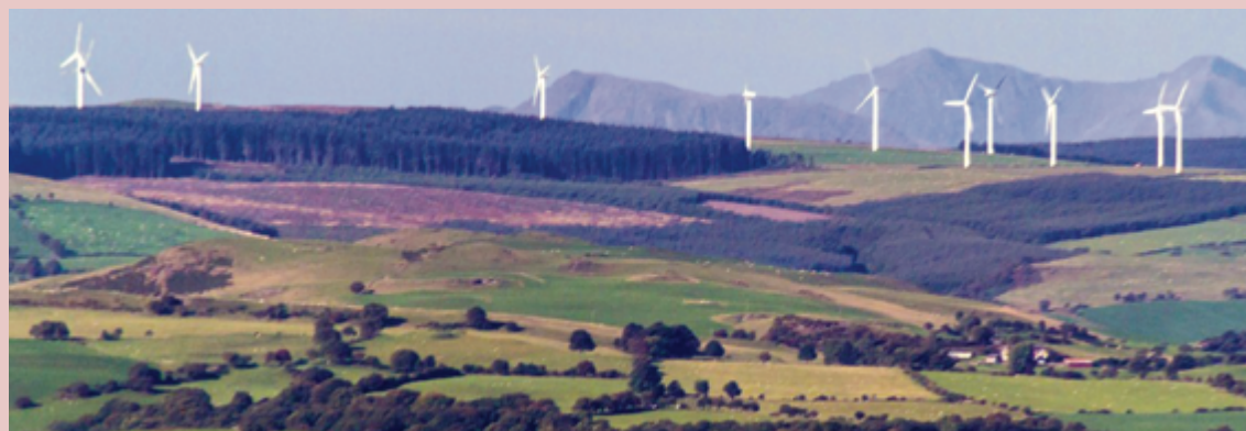
Tir Mostyn Wind Farm, North Wales. Photo: Peter McDermott
